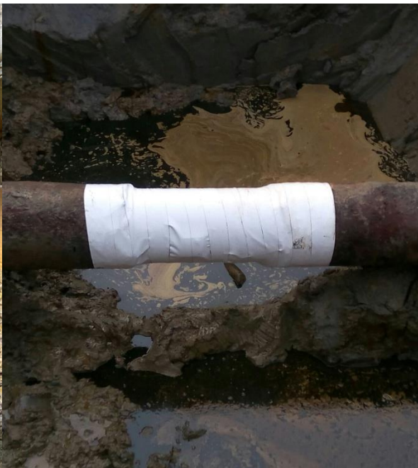
Spill point after repair
